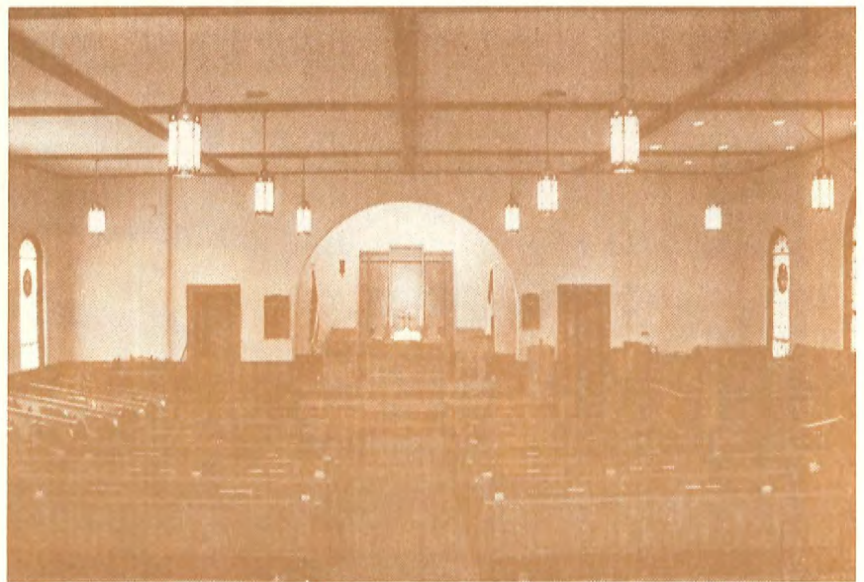
Sanctuary after renovation Completed in 1973
